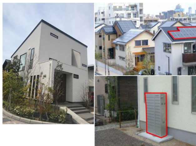
Fig 5-3 Appearance and energy system of the target residence
