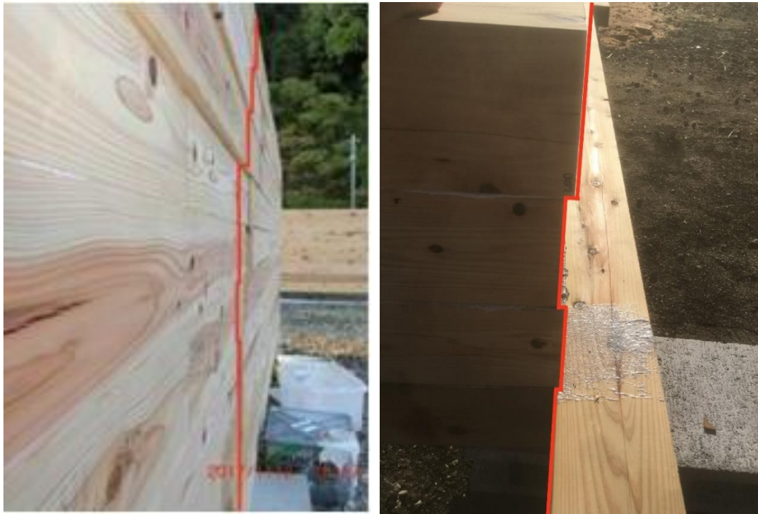
Fig. 6-13 Manual construction site photos.
