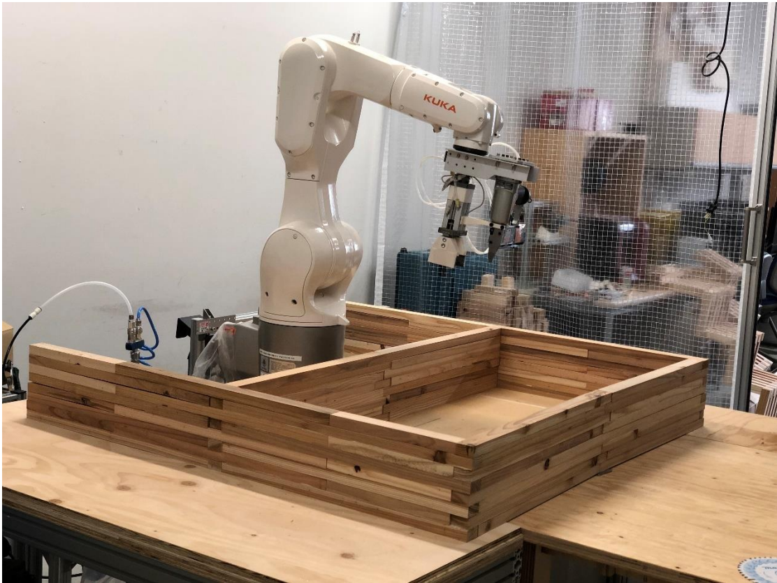
Fig. 6-18 Robot construction site photo.
