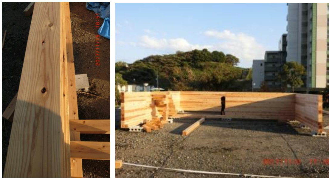
Fig. 6-14 Manual construction site photos.
