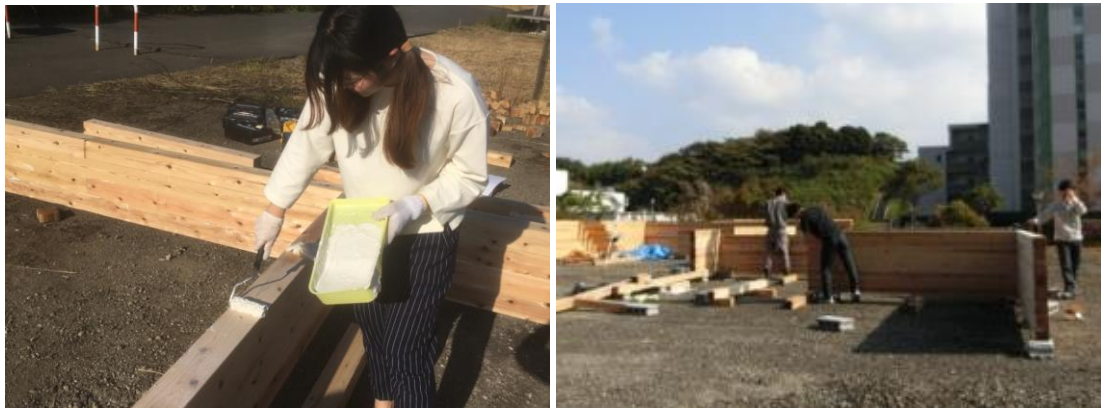
Fig. 3-11 Unit connection with glue and nail.
