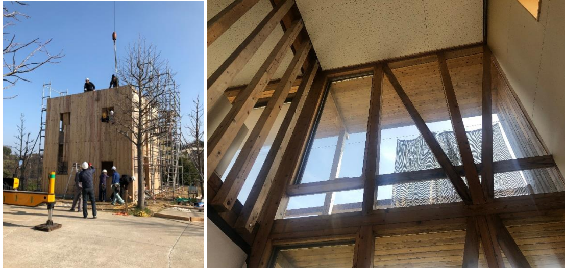
Fig. 3-5 Building construction site (left) and interior view after completion (right).
