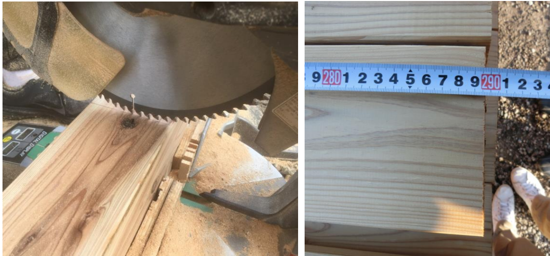
Fig. 6-11 Manual construction site photos.
