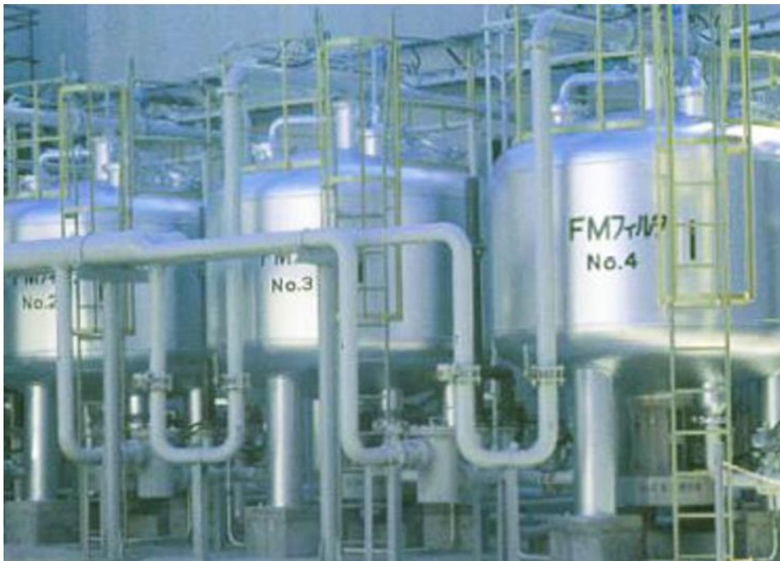
Fig 2-17 The FM filters in the rainwater subsystem of the HRG
