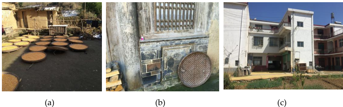
Figure 4-22. (a) Wall material for rammed earth structure; (b) Wall material of brick and wood structure; (c) Walls of reinforced concrete frame structures.
