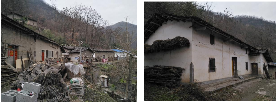
Figure 5-2. Photo of the present situation of folk houses in southern Shaanxi.
