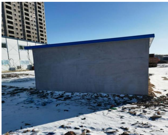
Fig4-5 East side of the laboratory room
