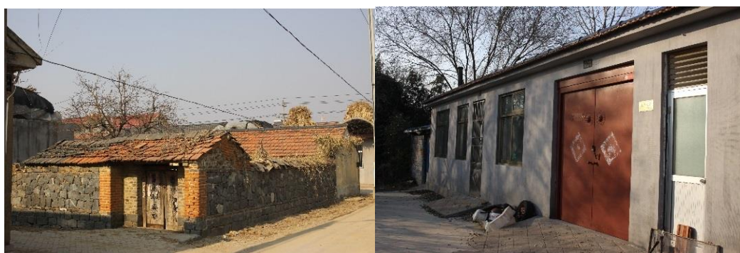
Figure 4.19 Abandoned house for all year and seasonal abandoned house
