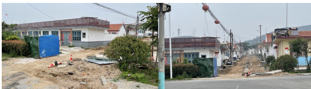
Figure 4.23 Common phenomena of unfinished construction
