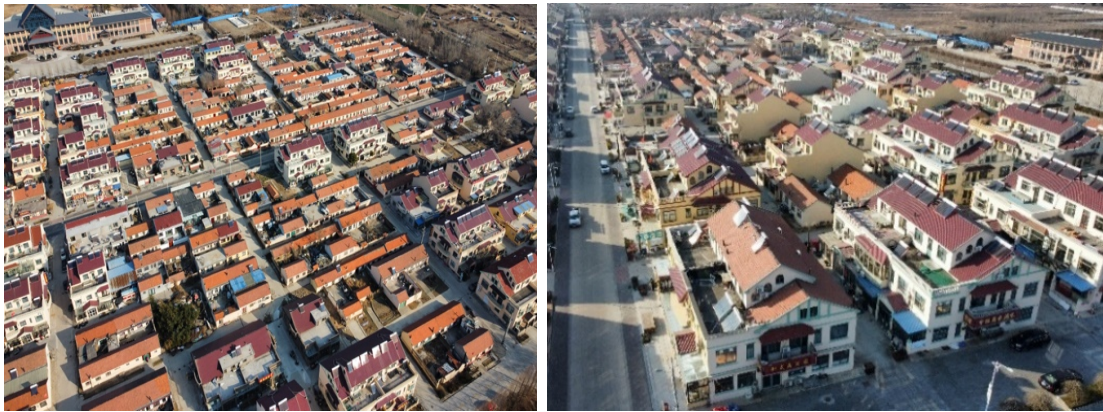
Figure 5.9 Modern vernacular dwellings in Wangjiataihou Village
