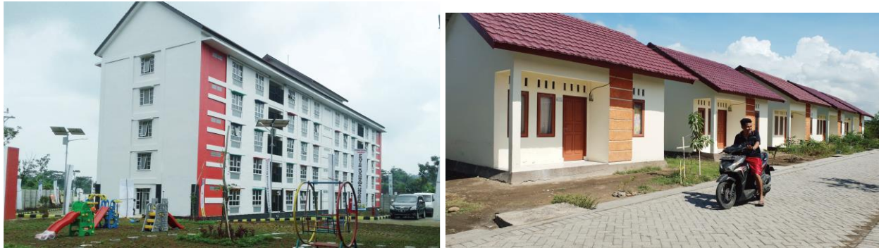
Figure 57. Vertical and Landed Housing for Low-income in Indonesia [371]
