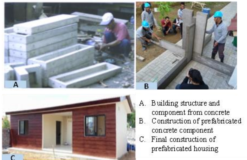
Figure 58. RISHA and RUSPIN: prefabricated concrete components for Low-cost Housing in Indonesia [284] [285] [286]
