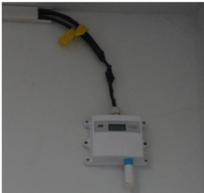
Fig 3-28 Indoor temperature and humidity sensor
