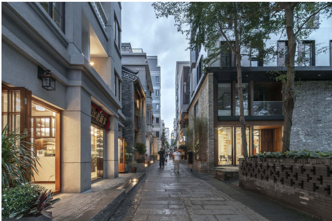
Figure 7-12. The main road after renewal.
