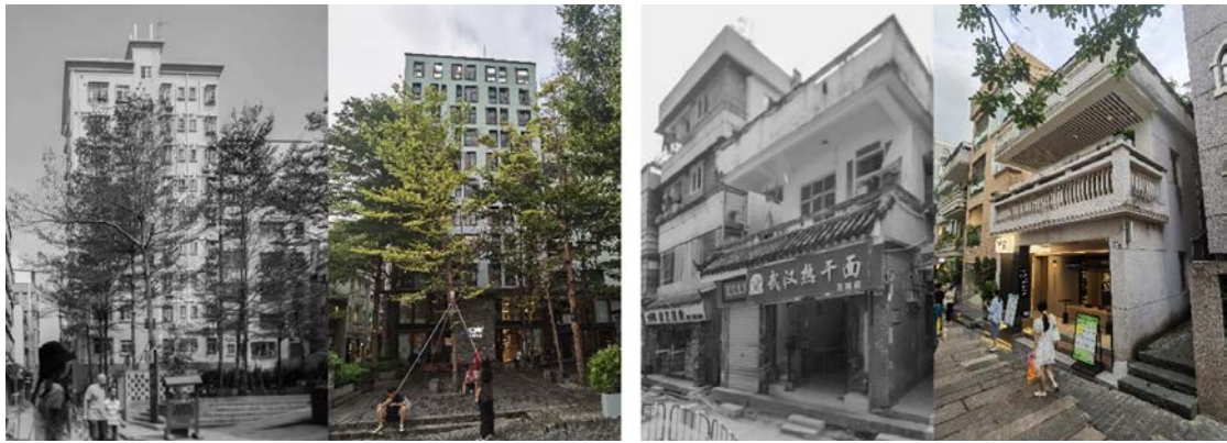
Figure 7-11. The original and new appearance of the renovated building
