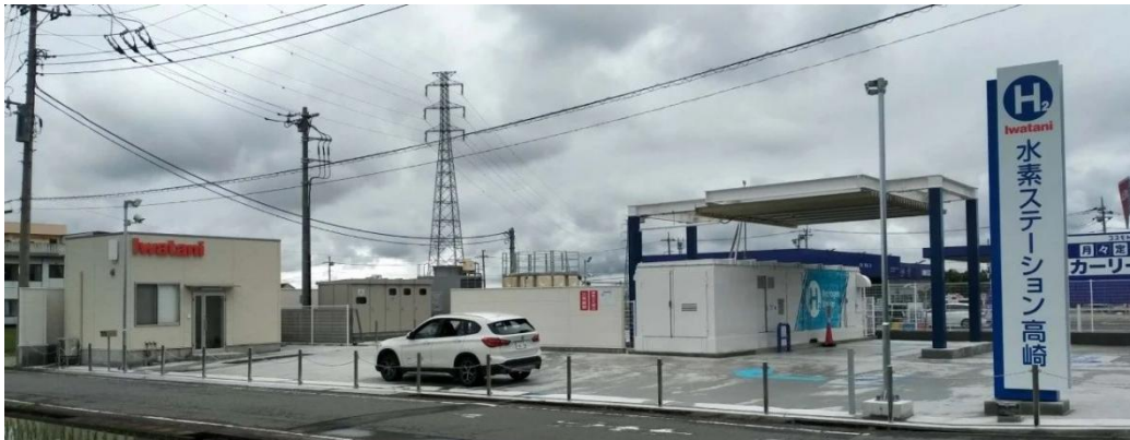
Fig.2-2 The overall structure of "Yamaguchi Hydrogen Station Gunma Takasaki"(イワタニ水素ステーション群馬高崎)[30]
