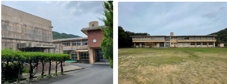
Figure 7-8 The original building and the view from the backside of the school building
