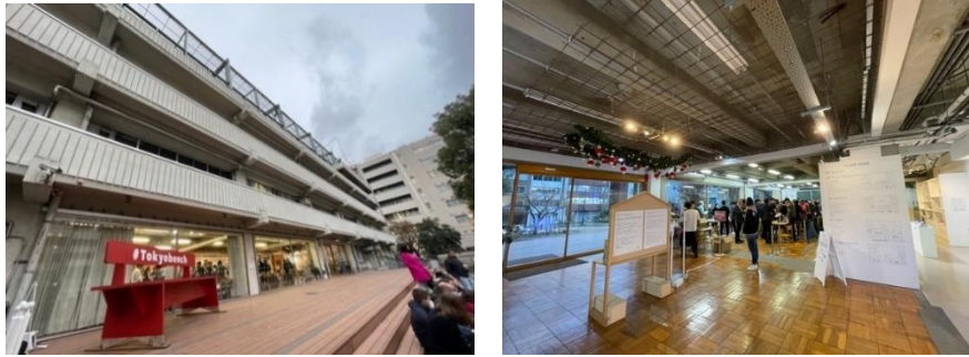
Figure 4-16 Exterior corridor (Left) and intermediate space (Right)
