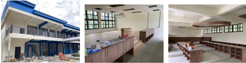
Figure 7-9 Overall space reconfiguration in checheng elementary school, Pintung, Taiwan
