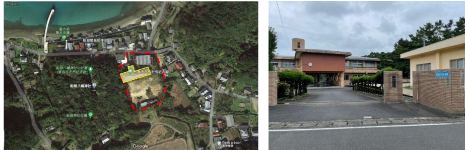
Figure 7-7 Aerial view of campus environment and the Funa-mawari Elementary School. Narushima, Goto City, Nagasaki Prefecture, Japan.
