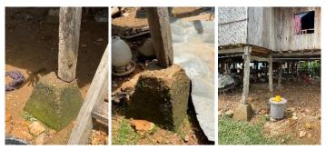
Figure 6.16 Columns placed on the cement blocks after the move
