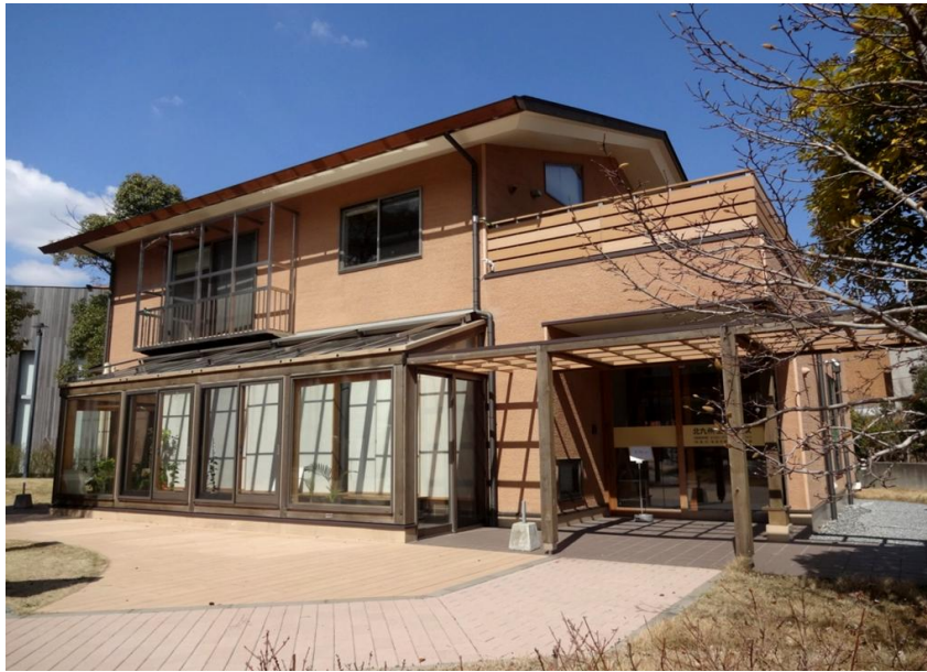
Figure 6-2 Physical appearance of Kitakyushu Eco-house
