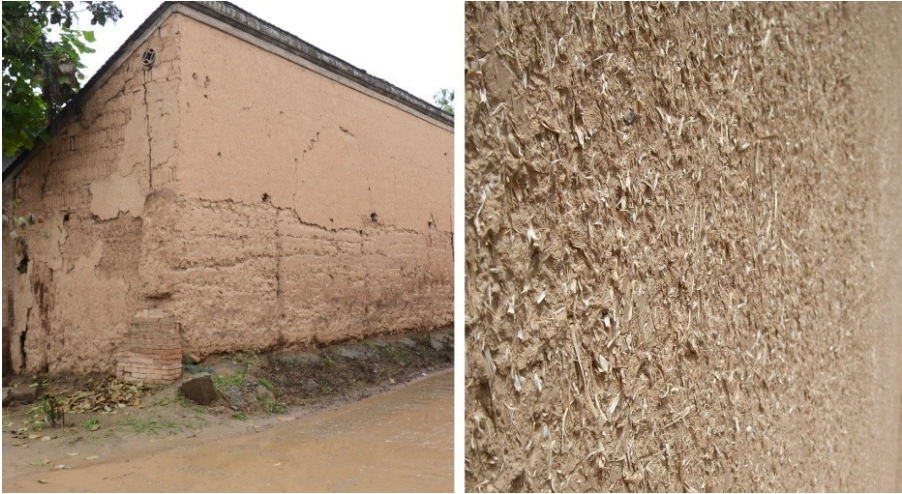
Figure 5.3 Wall made by immature soil
