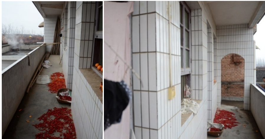
(a) West side of the second floor
