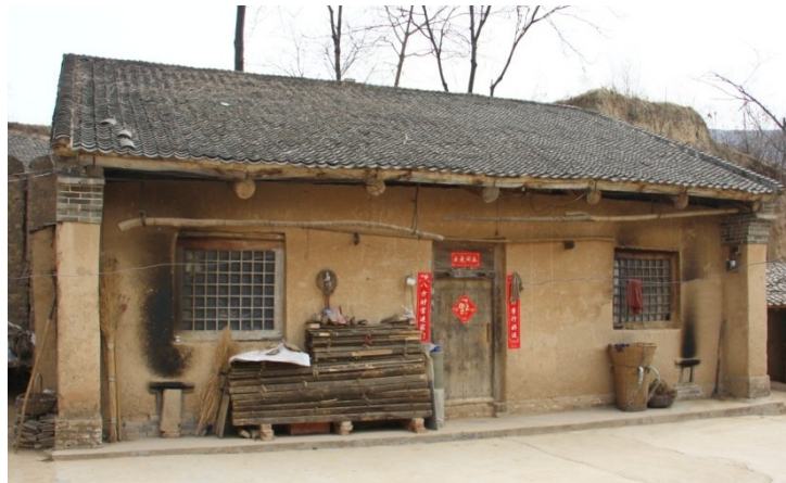
Figure 7.4 Present situation of the adobe residential building
