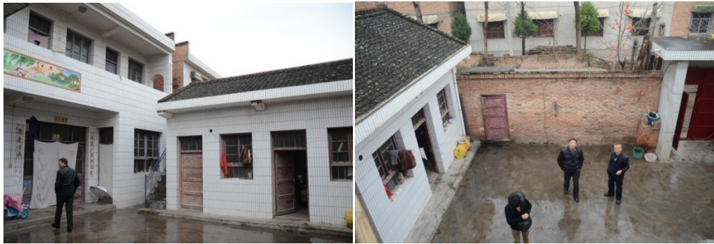
(a) East side of inner courtyard
