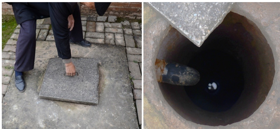
Figure 5.8 Existing water cellar in residential courtyard
