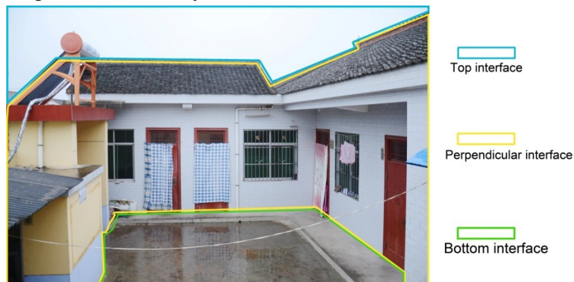
Figure 6.1 The composition of interfaces in courtyard of vernacular dwelling
