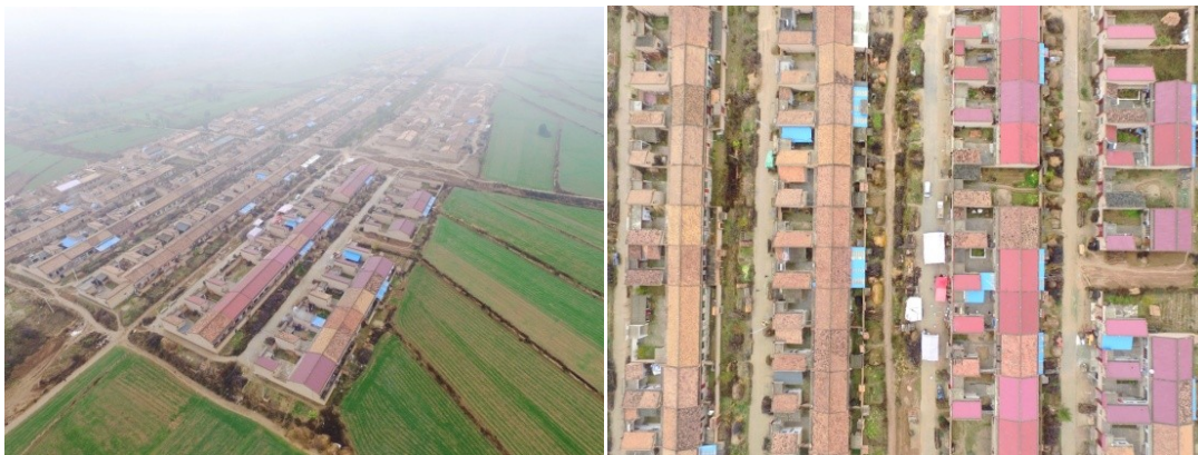
(a) Aerial view of the whole village (b) Aerial view of vernacular dwellings
