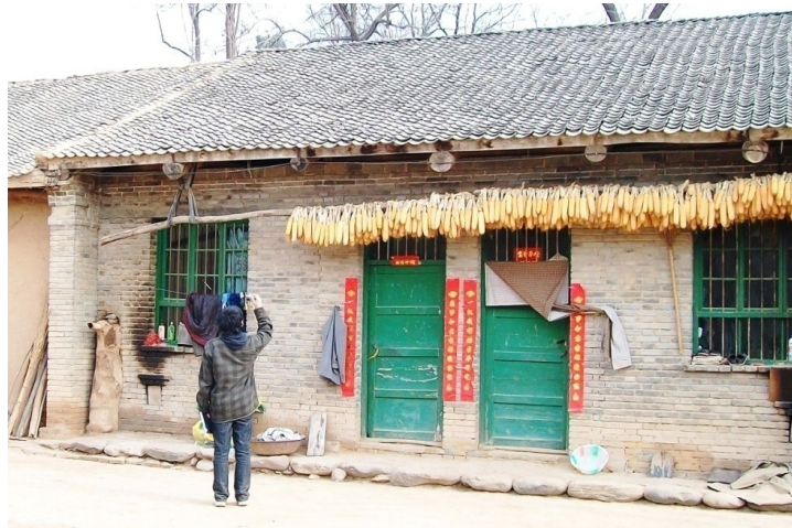
Figure 7.7 Present situation of one-storey brick-concrete structure building
