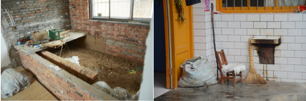
(a) "Kang" in the newly built vernacular dwelling (b)"Kang" entrance for adding fuels outside the room Figure 5.34 "Kang" is still kept in the newly built vernacular dwellings
