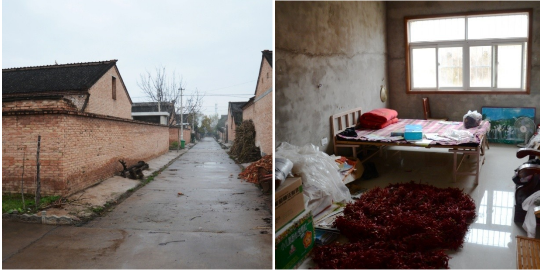
Figure 5.24 Poor quality of brick-concrete structure vernacular dwellings
