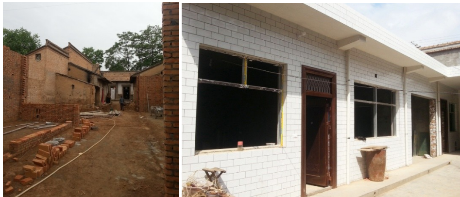
Figure 5.21 Construction site of brick-concrete structure vernacular dwellings in Qianyang County
