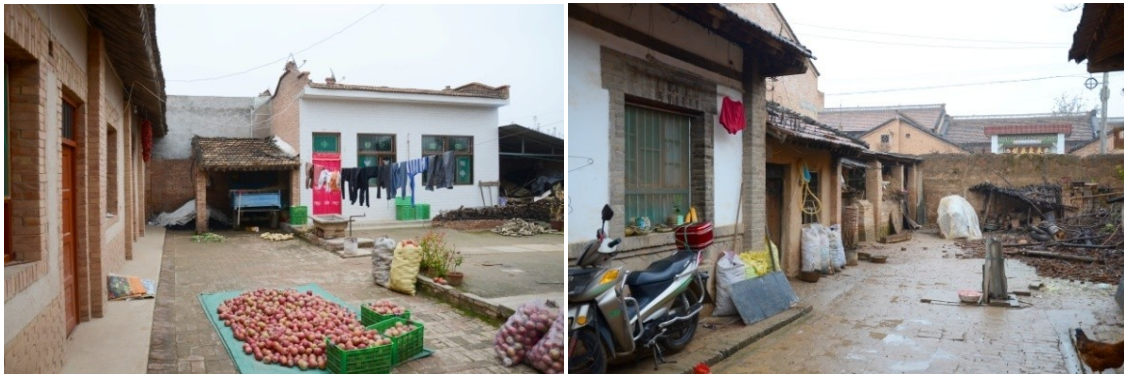
(a) Vernacular courtyard in Liang Jia Zhuang, Chun Hua County (b) Vernacular courtyard in Yu Jia Gong, Yong Shou County
