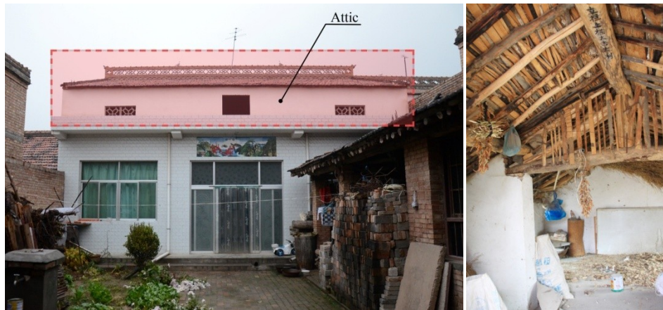
(a) Appearance of the attic
