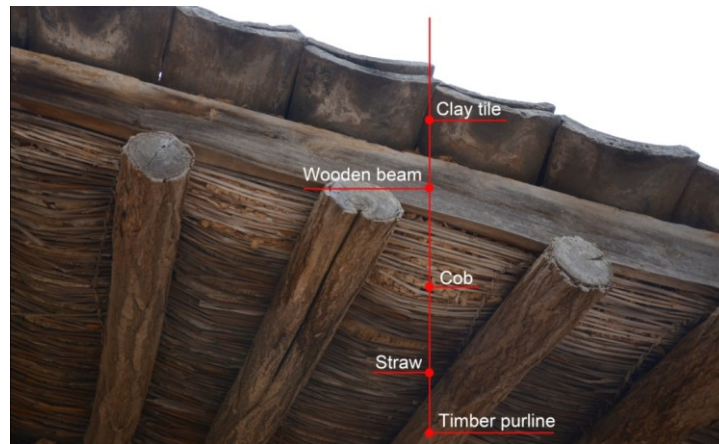
Figure 8.14 Roof construction of traditional residential building
