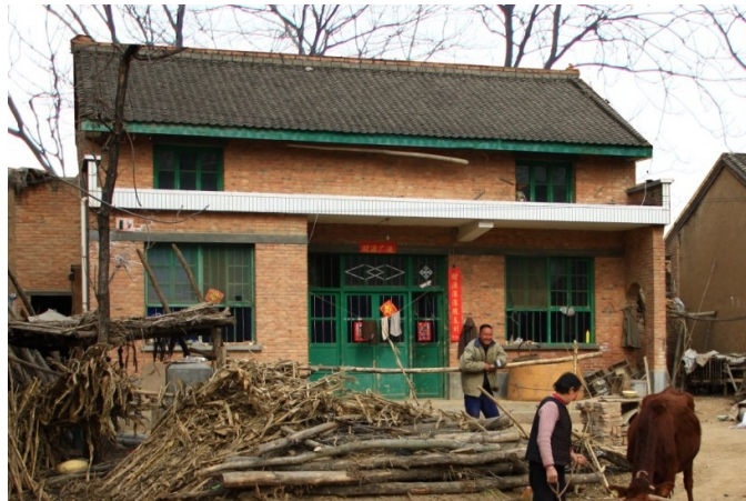
Figure 7.10 Present situation of two-storey brick-concrete structure building
