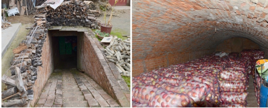
Figure 5.9 Existing soil cellar in residential courtyard
