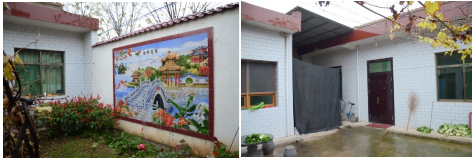
(a) East side of inner courtyard (b) South side of inner courtyard
