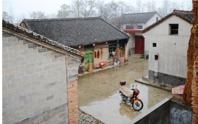
Figure 5.27 The dwelling that combination of adobe building and brick-concrete structure building in Yang Po village
