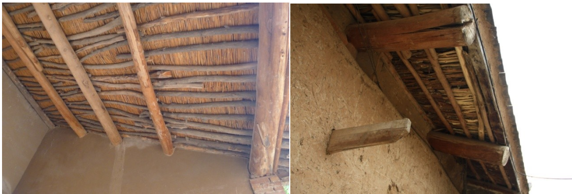
(a) Interior roof
