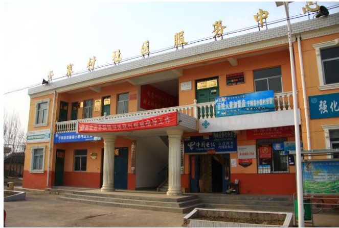
Figure 2.14 Government office buildings in Xiaozhai Village in Qianyang County
