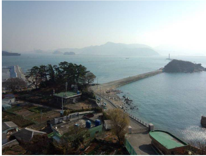
Figure 9: Busan New Port & Operation room
