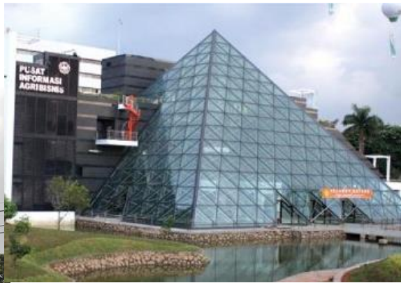
Source: (Admin n.d.) Ministry of Agriculture Building, Jakarta
