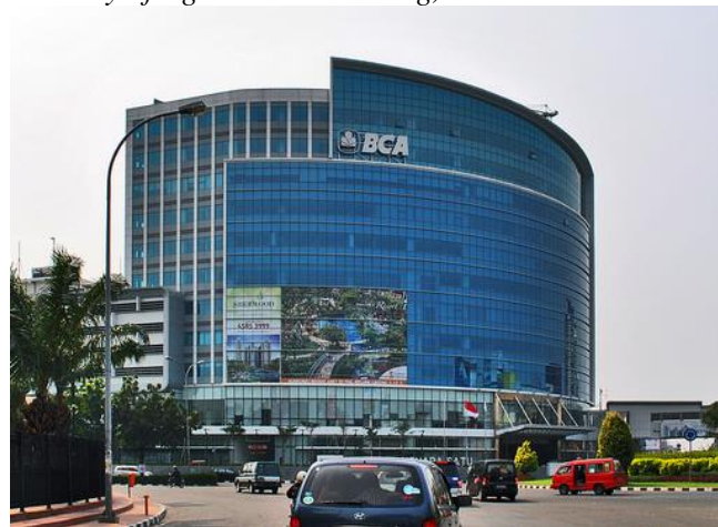
Source: Oka Sudiatmika Menara Satu building – Bekasi
