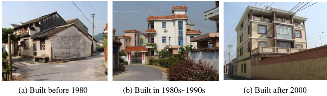
Fig.3-4 Rural houses of Pu'er village.
