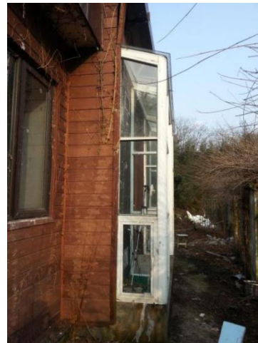
Fig.4-25. Trombe wall construction.
