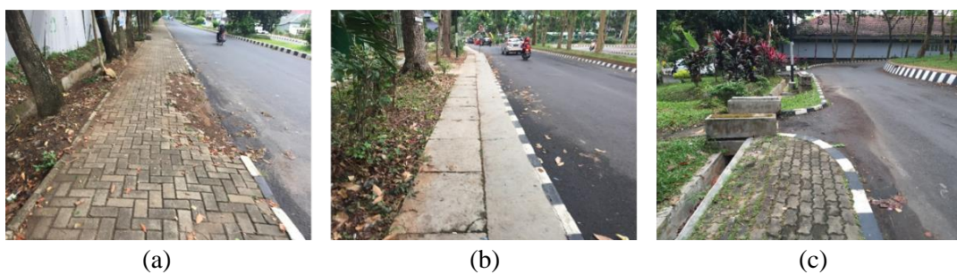
Figure 4.4 Dominant factors related to pedestrian dissatisfaction: (a) durability of path material; (b) aesthetics, (c) continuity of path without significant elevation differences.
