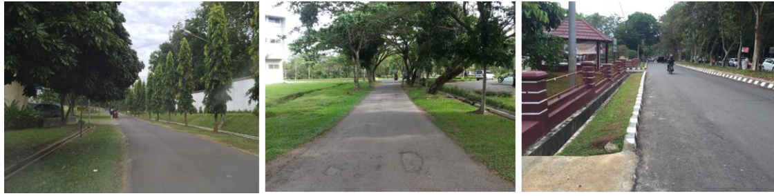
Figure 7.20 Existing conditions of sidewalks without lamps
