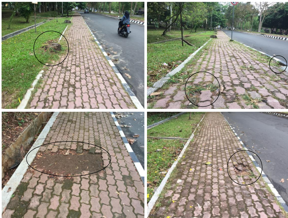
Figure 7.7 Existing conditions of UNILA sidewalks
