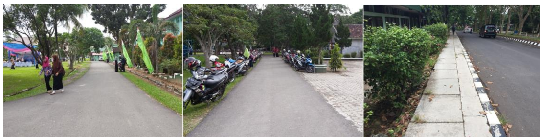
Figure 6.3 Narrow condition of sidewalks
