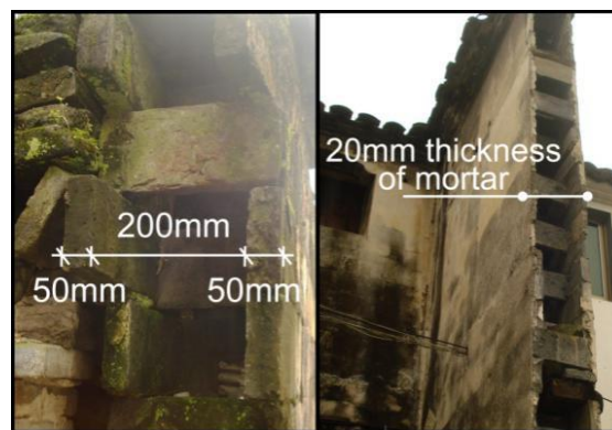
Fig. 8.1 Construction of the external cavity brick wall in Sizhai traditional dwelling
