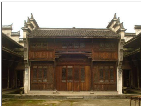
Fig. 4.11 External wooden wall in TPD in traditional dwelling
