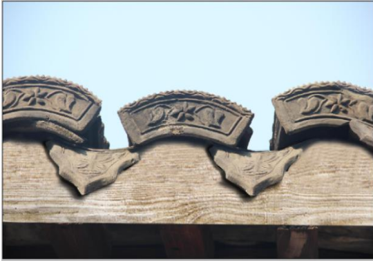
Fig. 4.13 Upward view of the roof details in traditional dwelling
