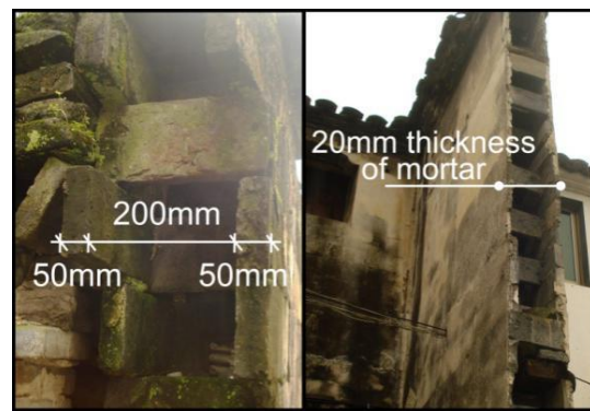
Fig. 4.10 Construction of external brick wall in traditional dwelling
