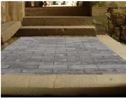
Fig. 4.17 Flooring on the first floor of traditional dwelling covered clay bricks
