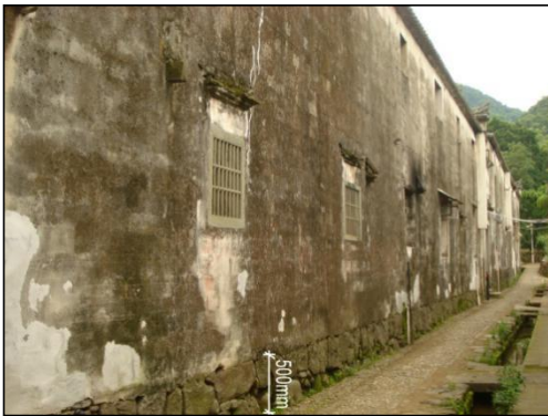
Fig. 4.9 External brick wall in TPD in traditional dwelling
