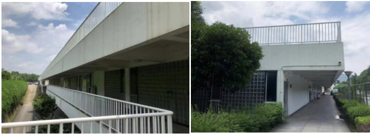
(7) Activity center and its entrances in YWICC
