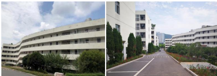
(12) Danguiyuan apartment and its entrances in YWICC
