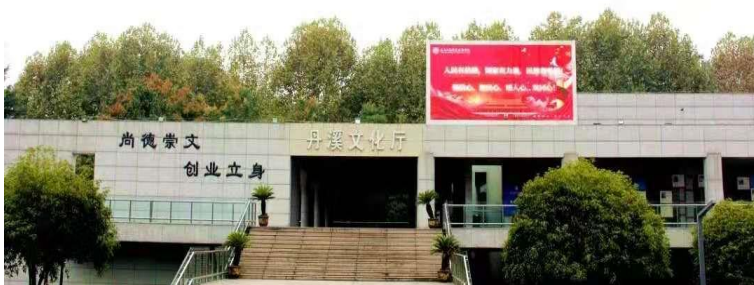
(14) Danguiyuan apartment and its entrances in YWICC
