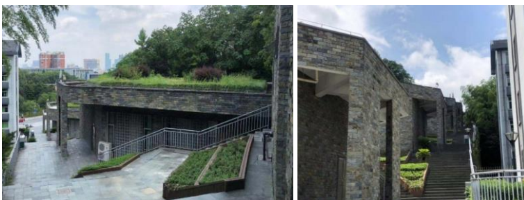
(8) Ladder promenade and its entrances in YWICC
