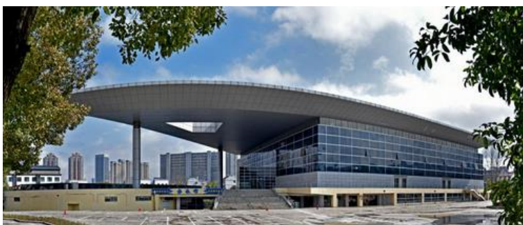
(4) Gym and its entrances in YWICC
