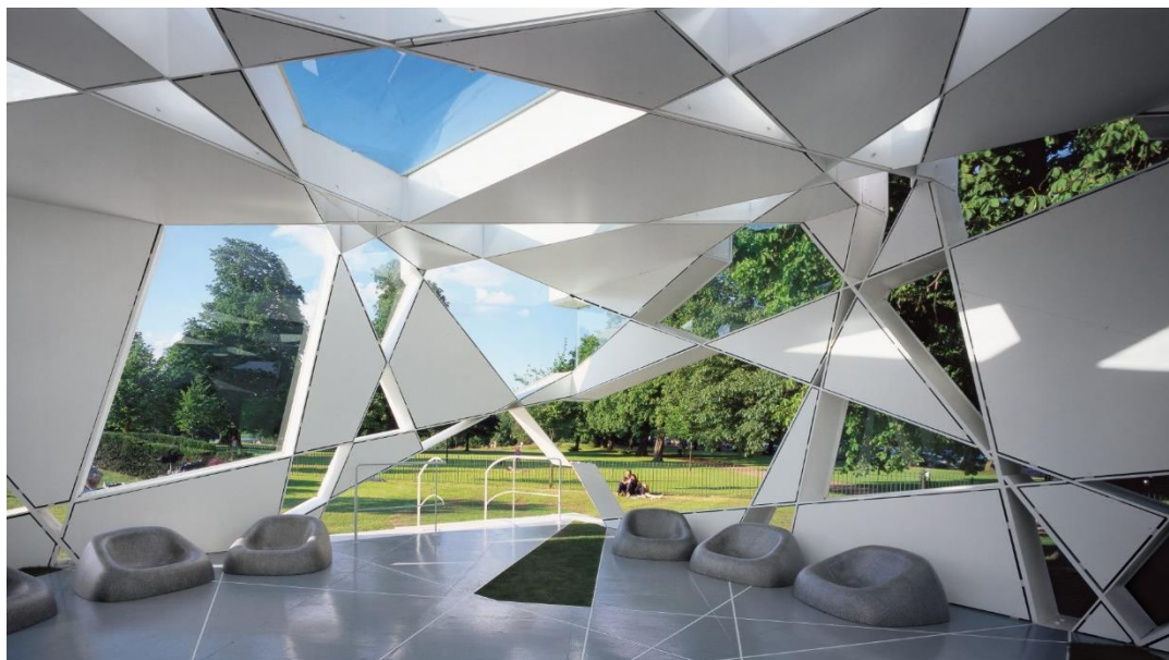
Fig. 17 - The Serpentine Gallery Pavilion 2002 by Toyo Ito and Cecil Balmond, appeared to be an extremely complex random pattern derive from an algorithm of a cube that expanded as it rotated.
