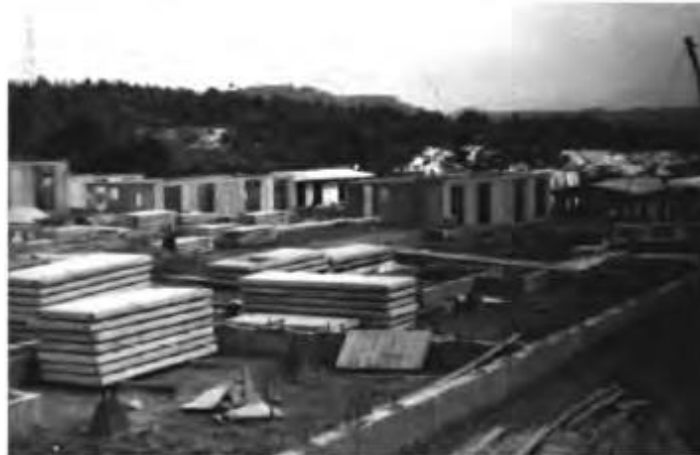
Figure 2.16. Toyota A-type Precast Concrete Building [44]
