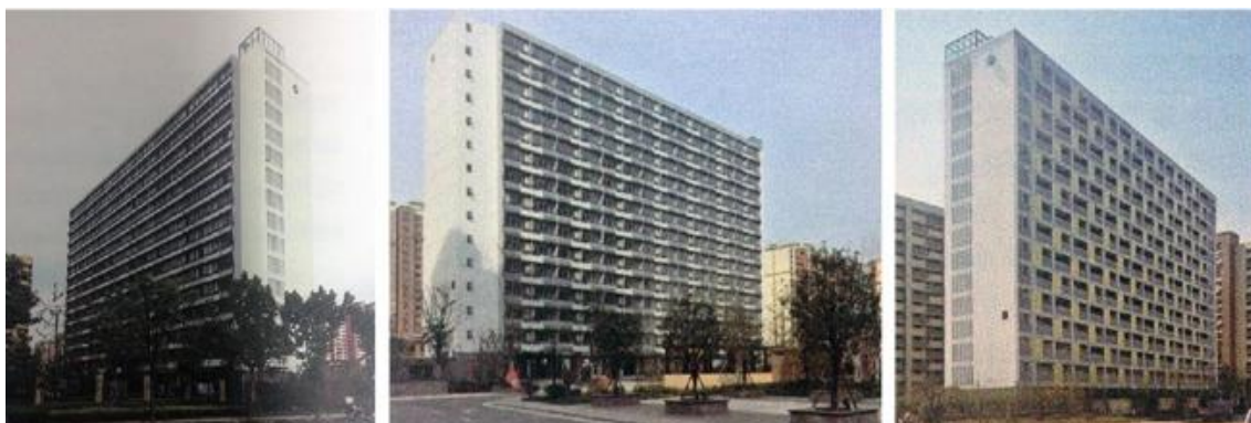
Figure 2.49. Nanjing Vanke Shangfang Affordable Housing Project [56]
