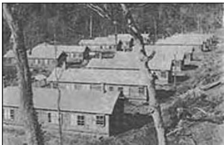
Figure 2.15. Prefabricated Industrial Plants, 1950 [42]
