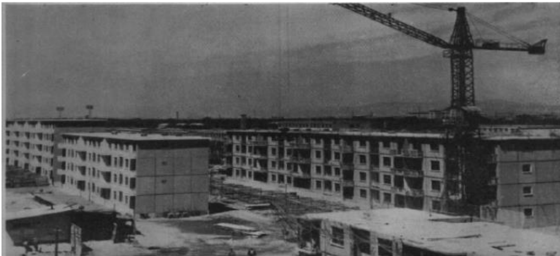
Figure 2.42. Beijing Tiantan Community under construction [50]
