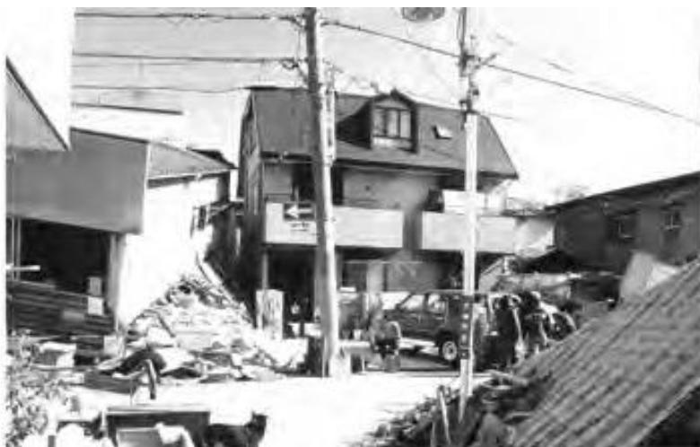
Figure 2.38. Prefabricated buildings after the earthquake
