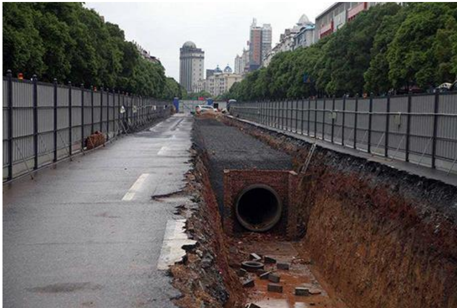
Figure 1.2 Open cut way for sewer pipe replacement project.
