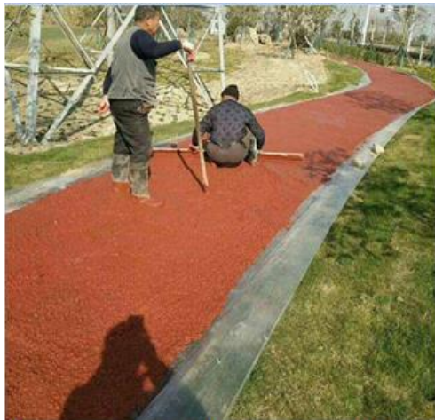
Water-permeable pavement (above)
