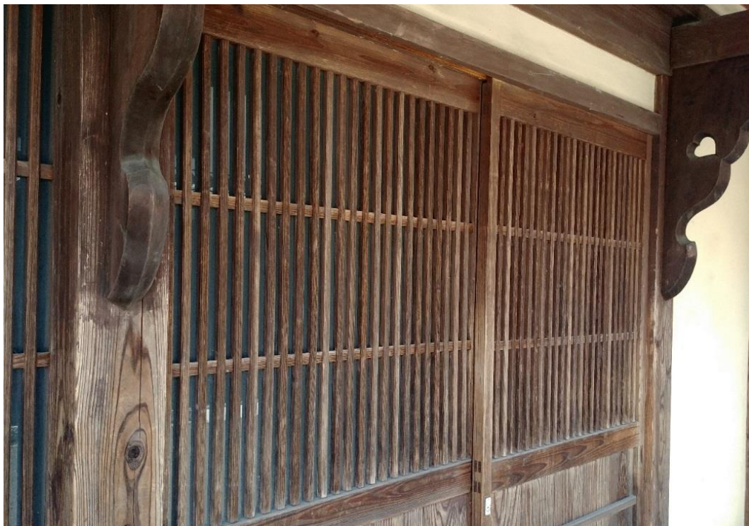
Figure 1. 32. Koshi is attached at the door frame.
