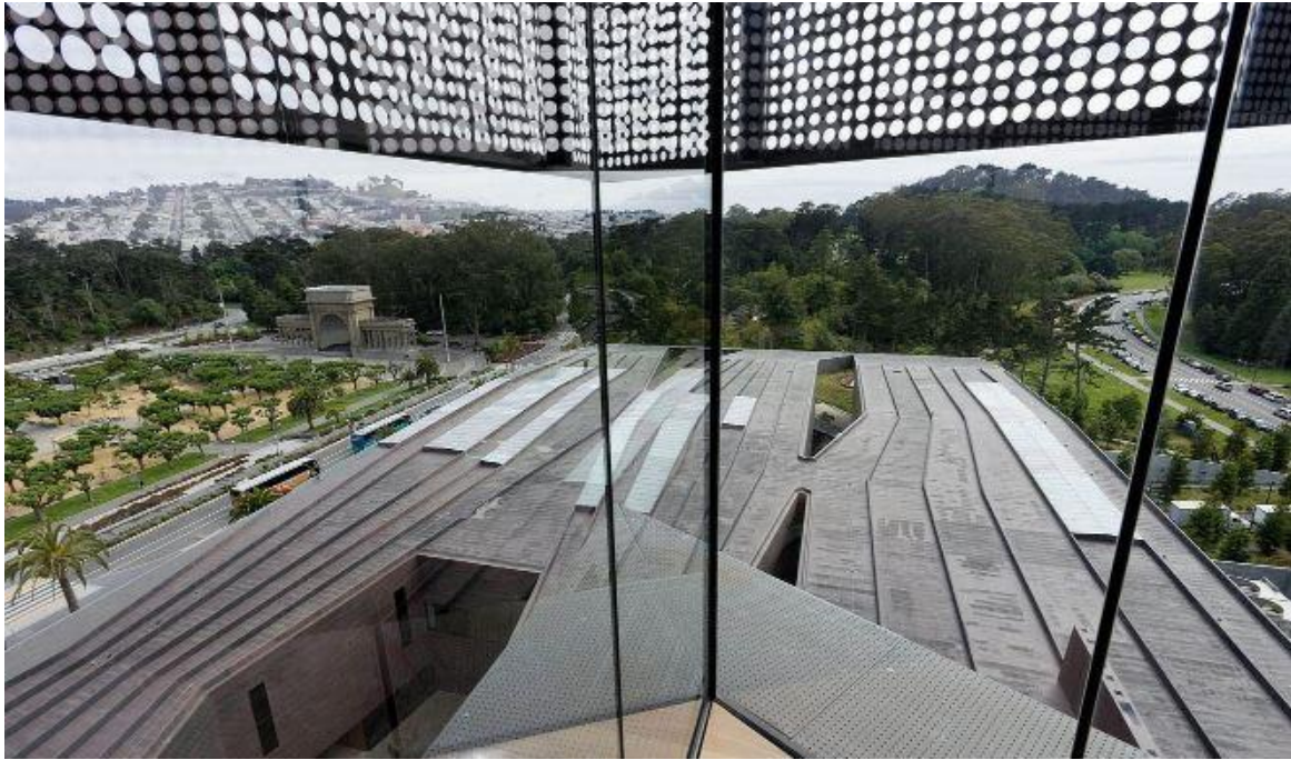
Figure 1. 38. Interior view of the perforated copper panel detail.
