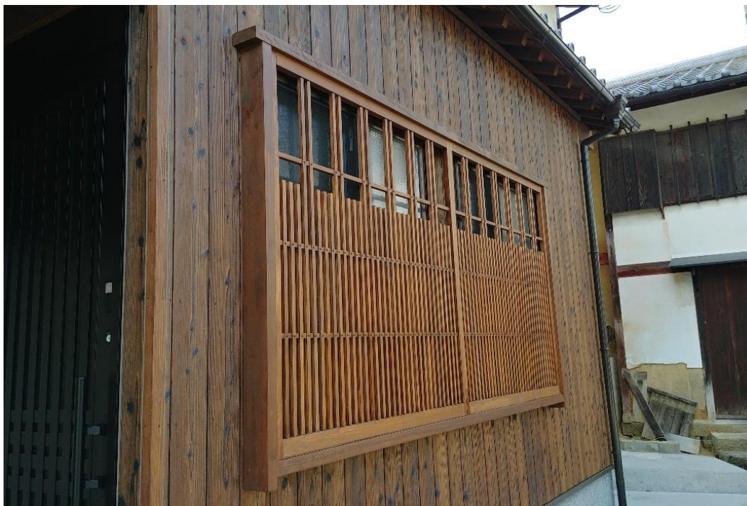
Figure 1. 33. Koshi is attached in the window frame.
