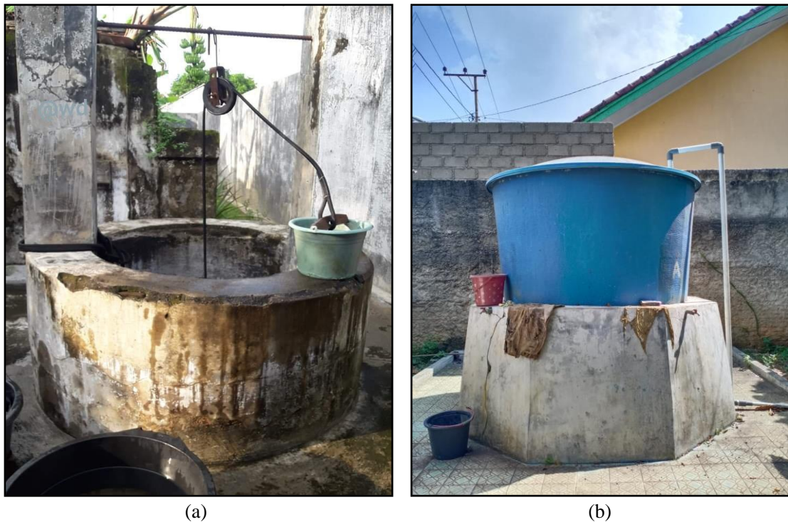
(a) Figure 4.6. (a) A dug well belonged to one of the residents of Kota Metro. (b) A communal bored well built by the government of Kota Metro
