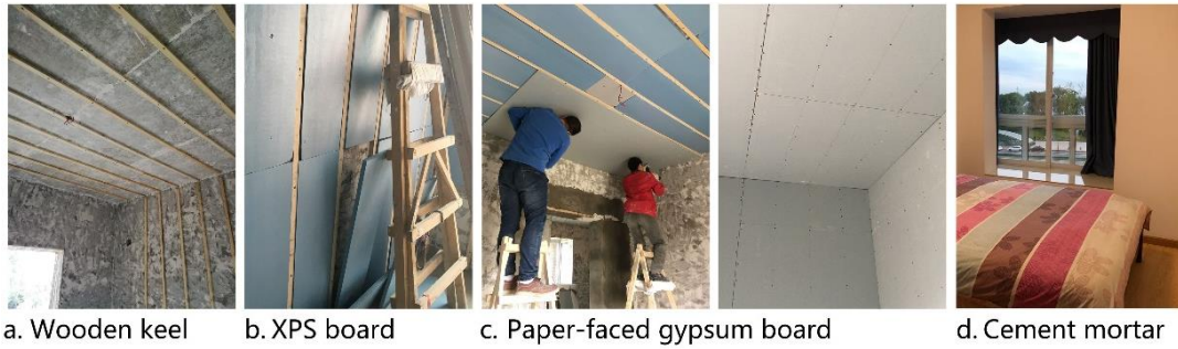
Figure 3-7. Overall view of the retrofit construction process.
