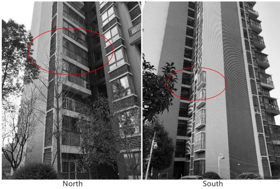
Figure 3-4. Overview of the selected residences: the original unit.
