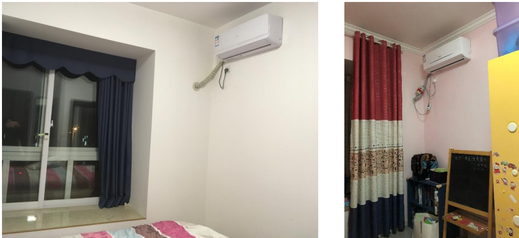
Figure 6-4. Actual view of the south bedrooms: renovated unit (left), and original unit (right).
