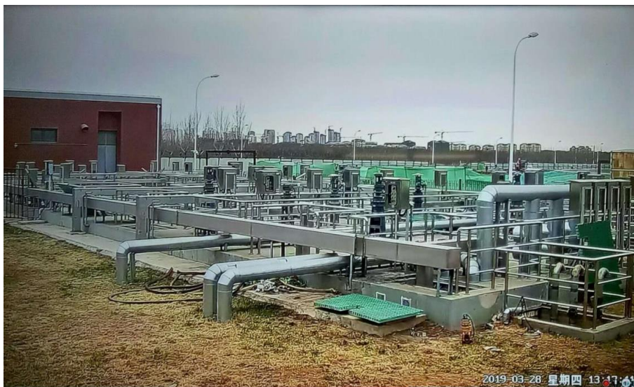
Figure 5.3a A view of Nankai WWTP’s structures (2019-03-28)
