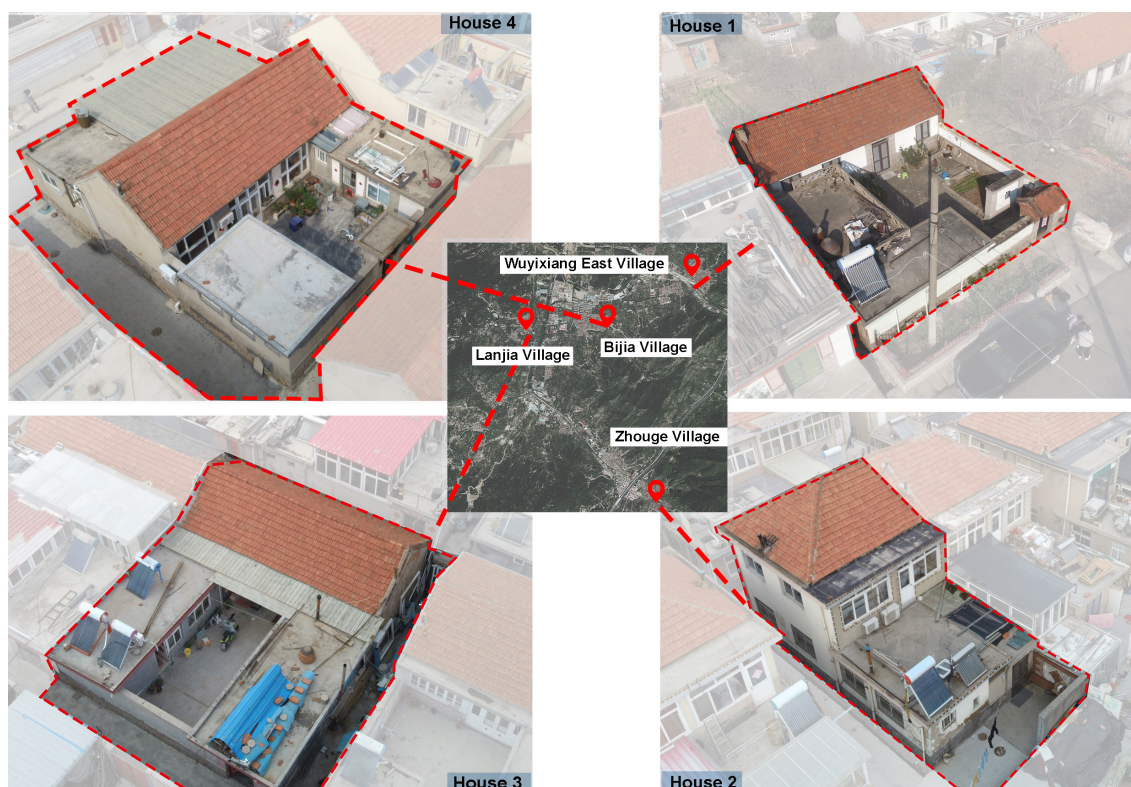
Figure 4.4. The location and photos of monitored buildings
