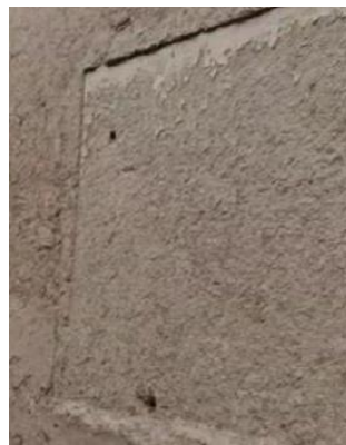
Figure 4-20. Rammed earth wall.
