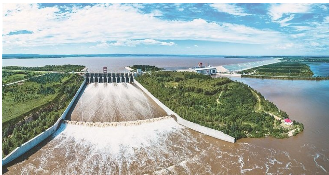
Fig.2-38 Nierji water control
