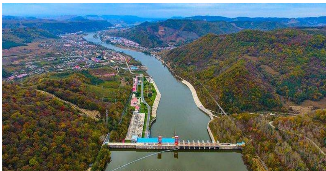
Fig.2-41 Hongshi hydropower station
