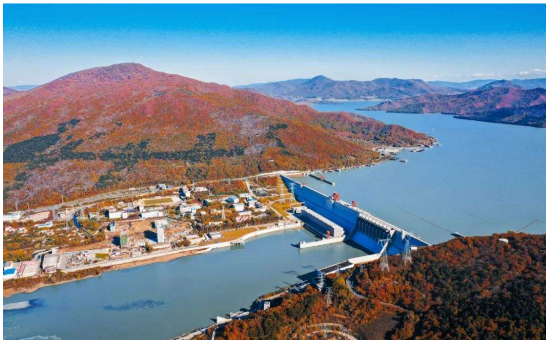
Fig.2-39 Fengman hydropower station
